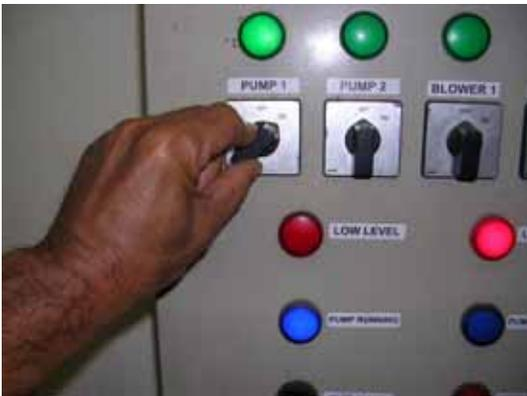
Pic12 Turn on the switch for the pump.
