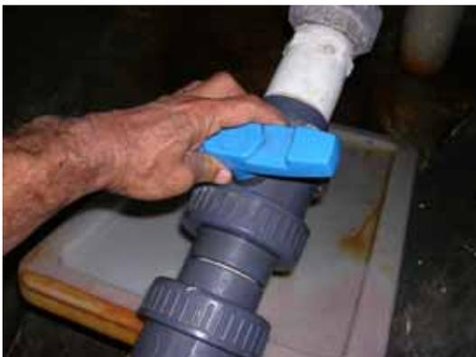
Pic5 Close the stop valve for the seawater intake pump.
