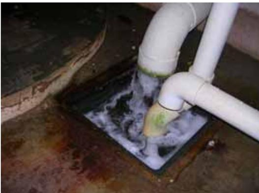
Pic3 Discharge of overflowed water. Now the tanks at the top of the pump house become full.
