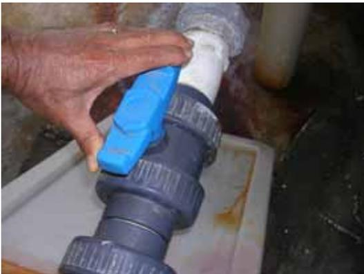
Pic11 Fully open the stop valve for the pump.
