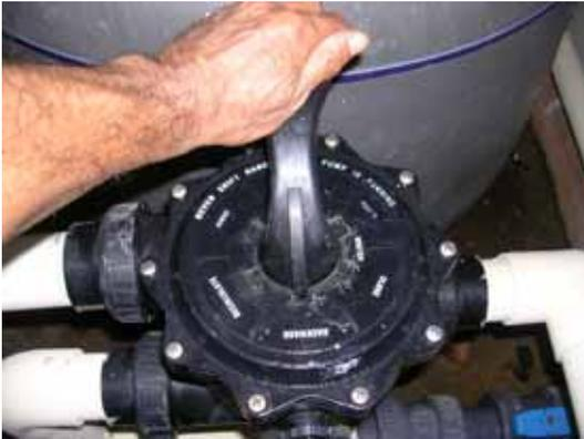
Pic10 Select the backwashing mode in the sand filter controller.
