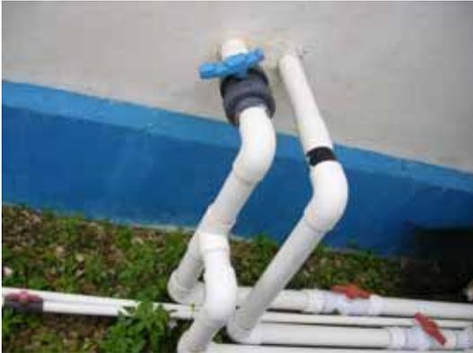
Pic1 The main valve (w/ blue handle) is located outside the pump house.
