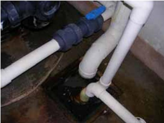
Pic2 4" drain pipe from the elevated water storage tanks appears in the center of this picture taken at the water discharge pit.
